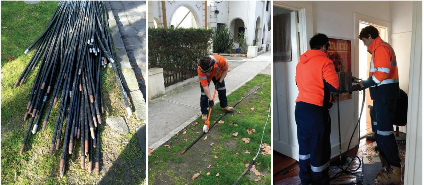
Above, left: An array of PowerPiles. Above, middle: A PowerPile is prepared for placement. Above, right: Retro-fitting of PowerPiles from inside the building.
