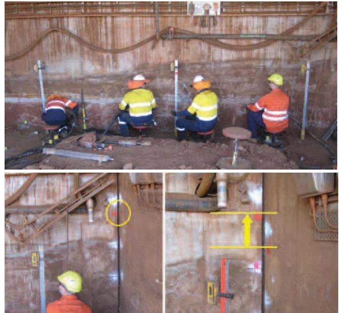
Above: Injection of resin simultaneously at 4 points.
