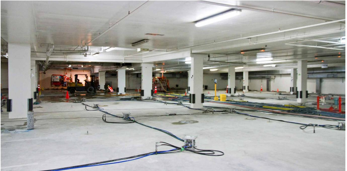
Above: Our JOG computer-controlled levelling team hard at work. The automated, neat, clean and quiet scene with progress of levelling monitored by sensors throughout the basement and observed in real time by our control room staff.
