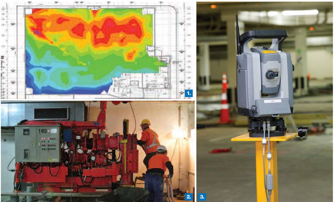
Pictured above: 1. Example of the continuous scanning of levels. The colours change constantly showing the progress of levelling in each area. 2. Our technicians operating a jet grout injection machine. Note the low head-room. Our smaller machines can create large soil-crete columns from much smaller rooms. 3. Our JOG computer-controlled levelling is monitored by sensors throughout the basement.
